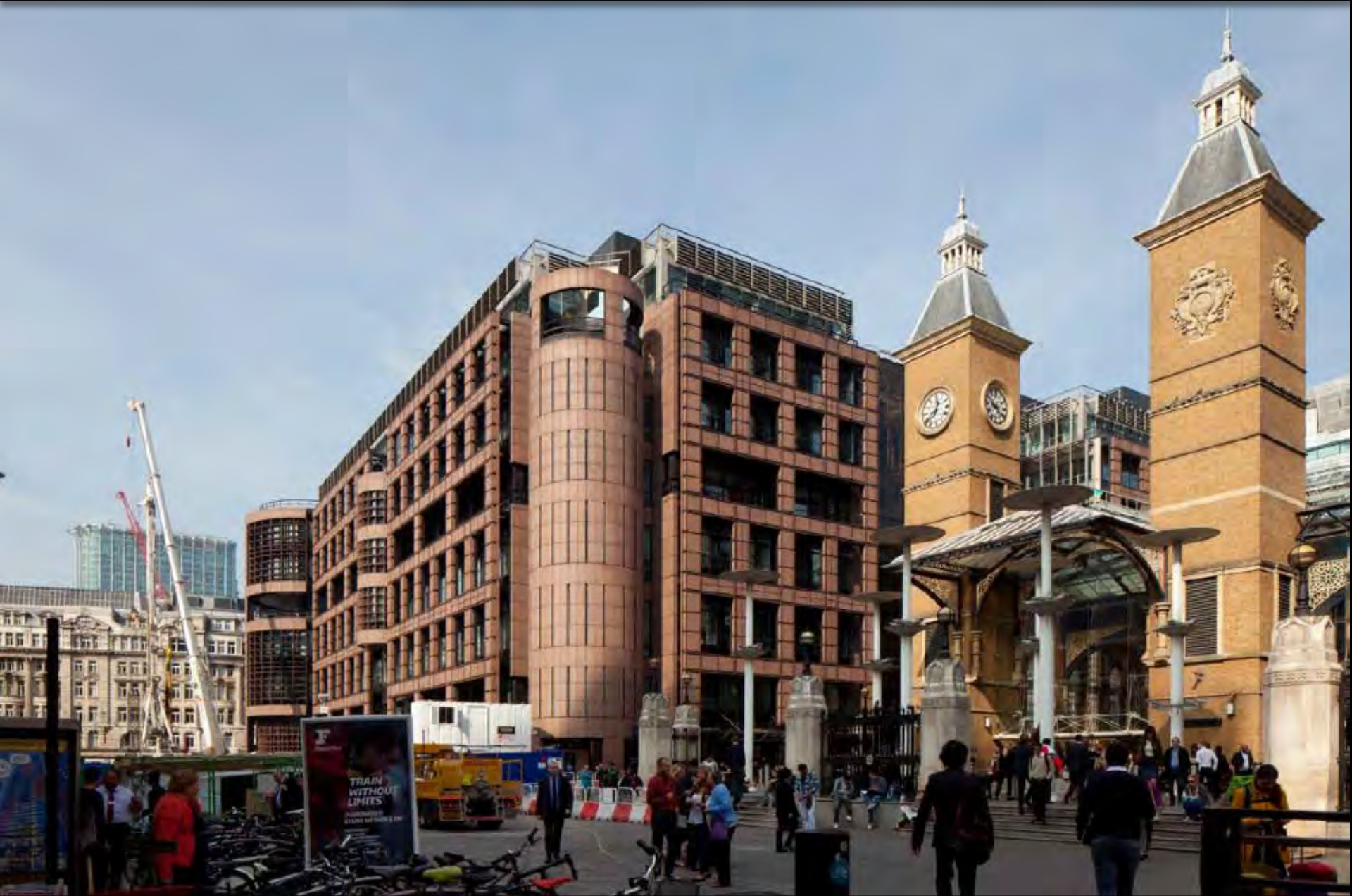
Existing view from Liverpool Street looking north-west
