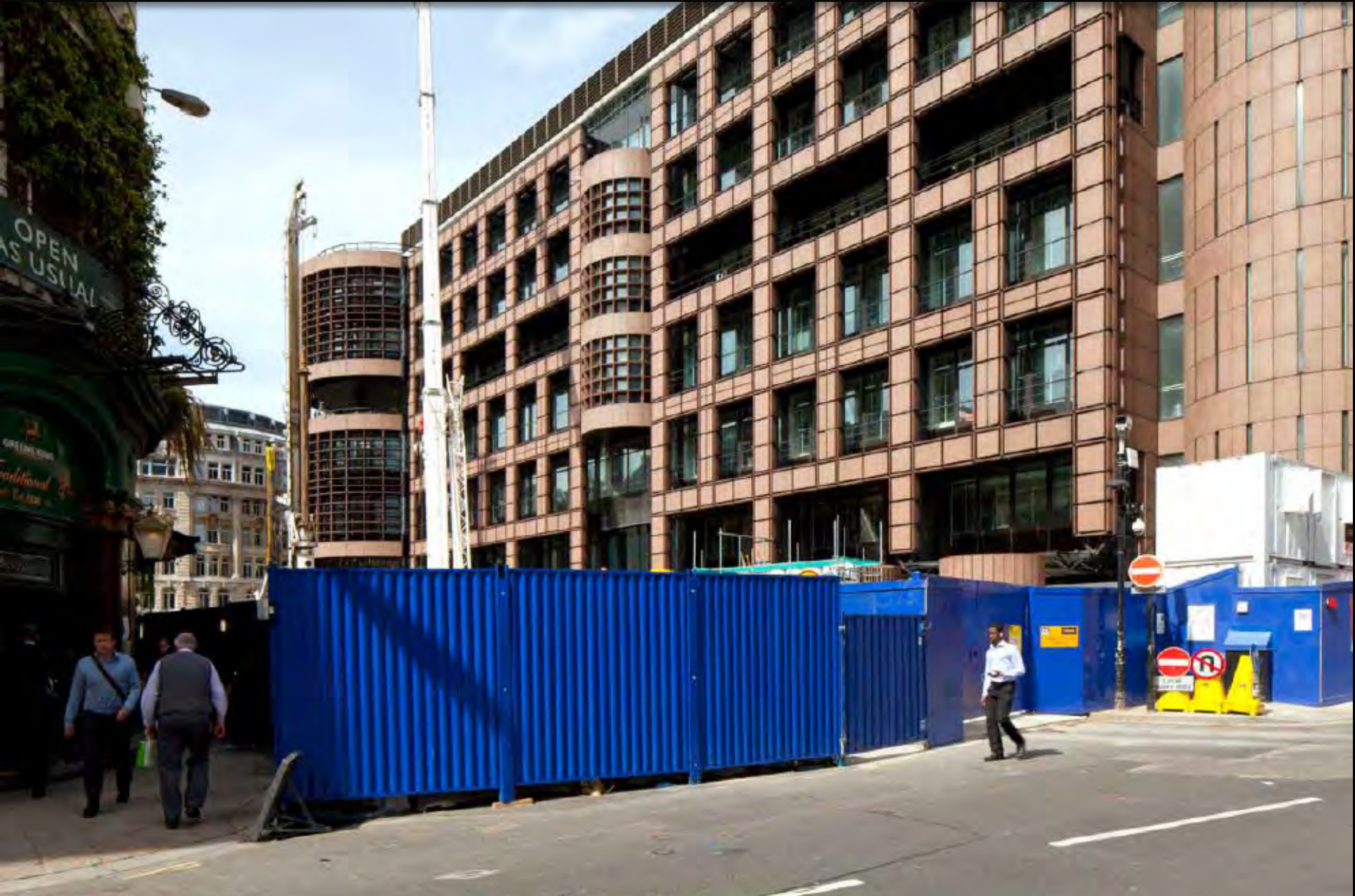
Existing view from Liverpool Street looking north-west
