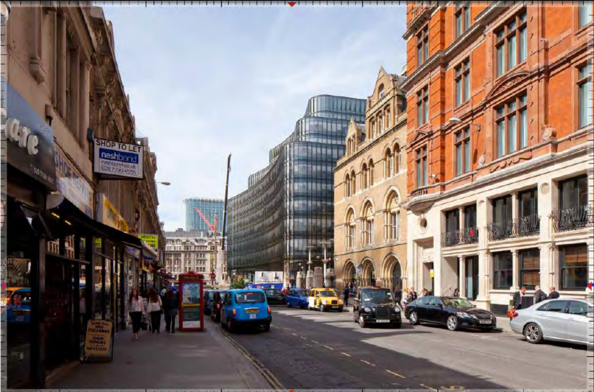
Proposed view from Liverpool Street looking west
