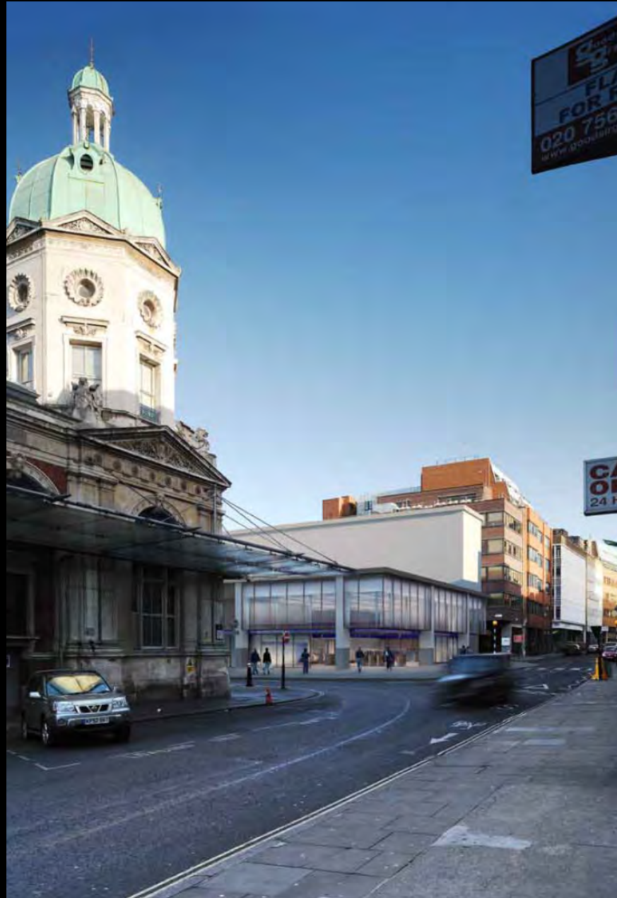
Long Lane, at the corner of Rising Sun Court, looking north-east
